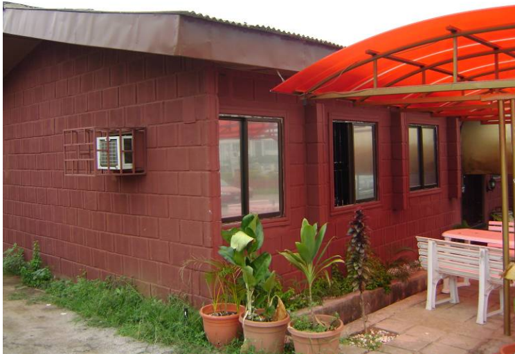
Fig. 1: Alagbaka shopping arcade built with Ire Burnt Brick, Akure, Nigeria (Photo <c> Adedapo Adebayo.)
