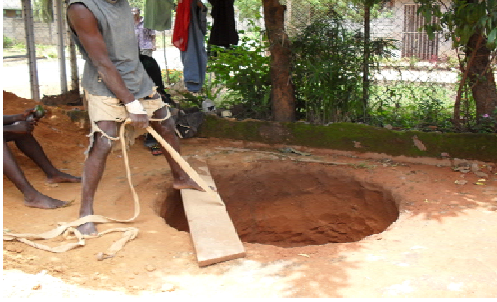
Figure 7: Deep Well Digging in Old Mabvuku.
