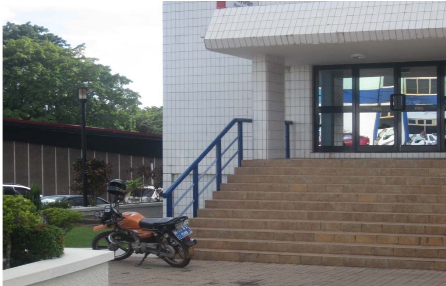
Figure 1: Entrance of a public building with no ramp provided
