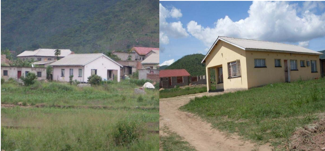
Plate 3 & 4: Houses built in Zimta and Z.H.F
