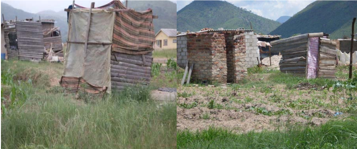
Plate 1 & 2: Outside toilets built with substandard materials
